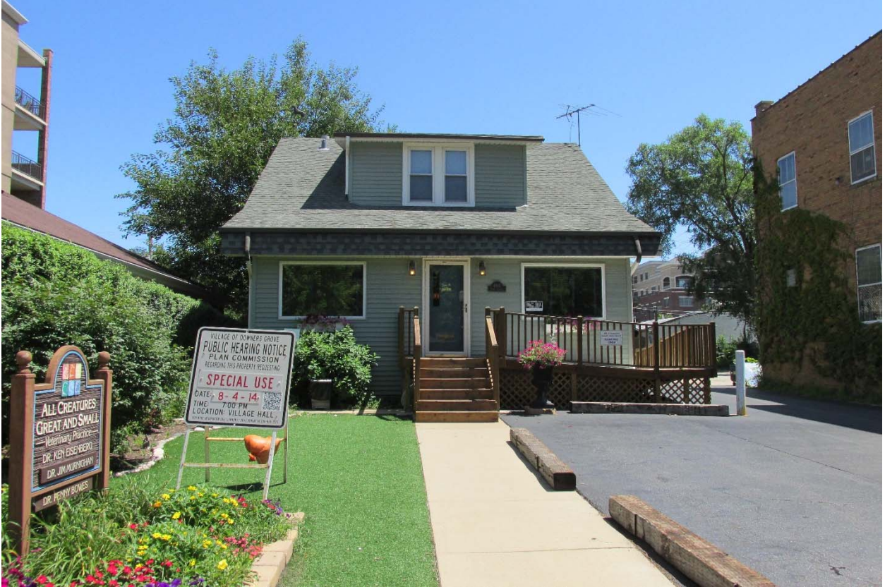
Figure 1 - Photo of the west elevation of the subject property.
